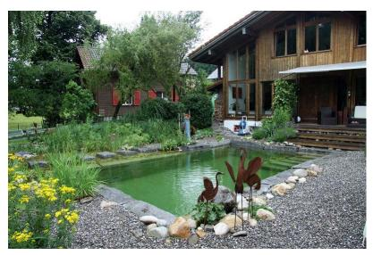
Natural swimming pools are built in either one- pot or two-pot designs. In one-pot designs, the regeneration zone is contained within the same chamber as the swimming area. The water flows over the top of a shallow retaining wall between the two areas.
