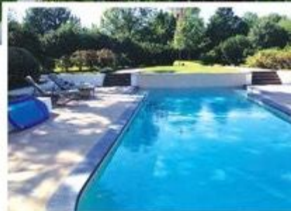
Allison Landscape & Pool Company converted an outdated pool (below) into a functional space (left).
